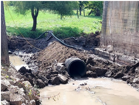
Pipe installed between footers. 15 holes drilled.
