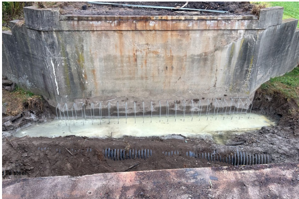
Cut rebar and tie steel
